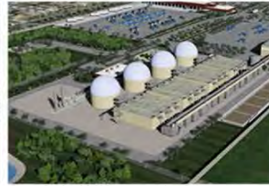
Anaerobic Digestion Facility - ADF
