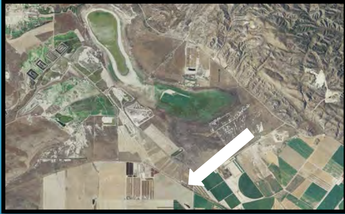
Breached Levee Location
