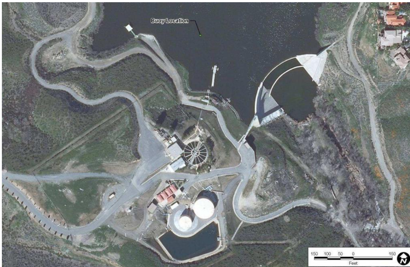
Figure 7: Buoy Location for Submerged Equipment
