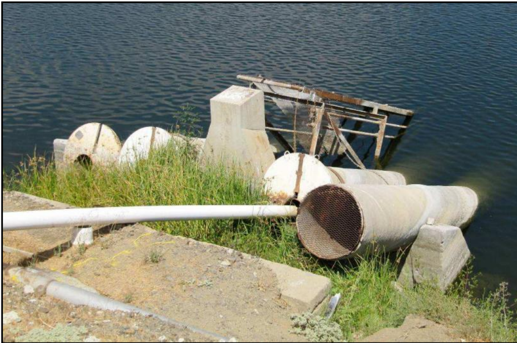
Figure 27: Abandoned Intake Structure and Pipes (Location B)
