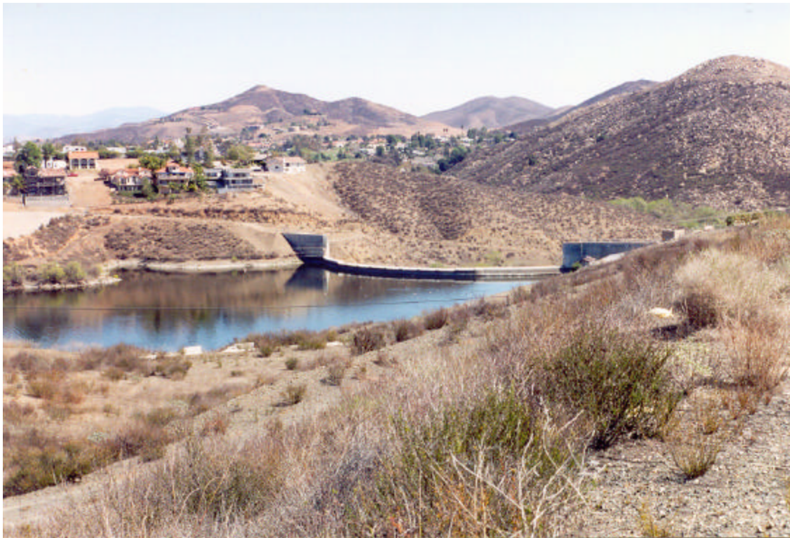
Figure 2-12. Canyon Lake dam – facing southeast
