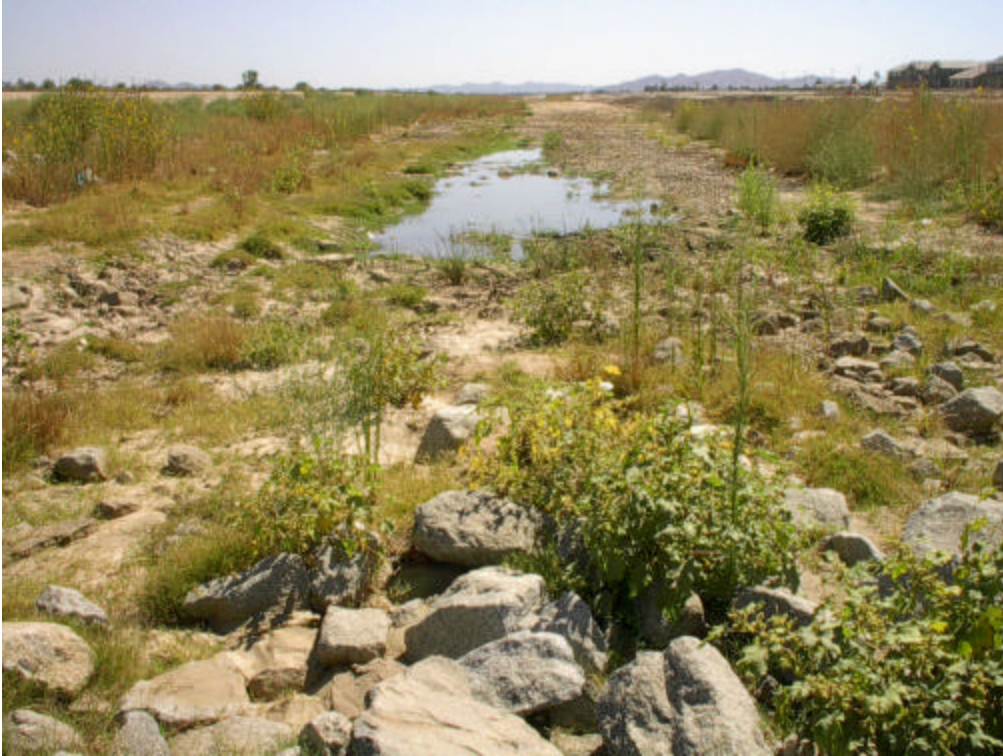
Figure 4-13-5. Perris Valley Storm Drain at Orange Street (looking downstream)
