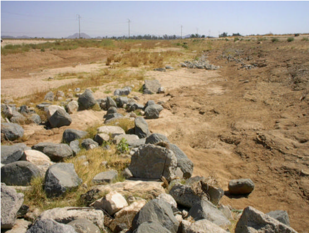
Figure 4-13-4. Perris Valley Drain at Rider Street (looking downstream)
