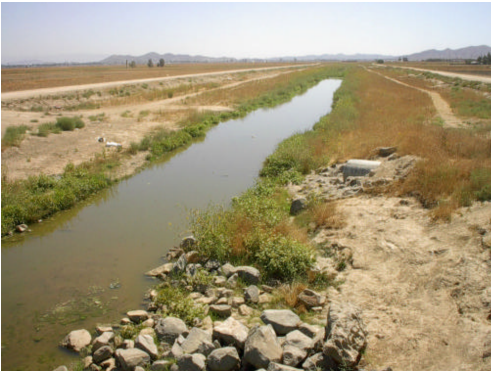
Figure 4-13-6. Perris Valley Drain at Nuevo Road (looking downstream)
