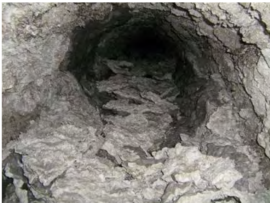
Figure 2-3 EMWD Pipe with Encrusted Scale
