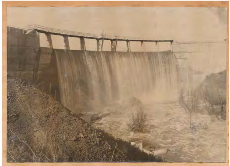
Figure 2-13. Overflow of Canyon Lake Dam, approximately 1936-1937 (Source: Lake Elsinore Naval School)
