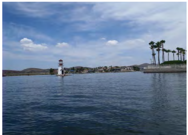
Figure 2-2. Canyon Lake Reservoir, 2016 (Source: Amec Foster Wheeler)
