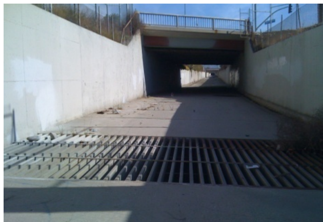
Figure 6 Automated Inlet located within San Antonio Channel Diverts Dry and Wet Weather Runoff to Montclair Basin No.1
