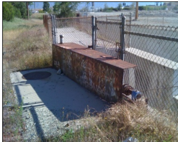
Figure 5 Outfall Diversion Structure to Montclair Basin No.1
