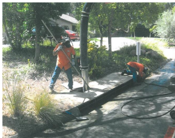
Figure 3-16. Catch Basin Cleaning in Riverside County MS4
