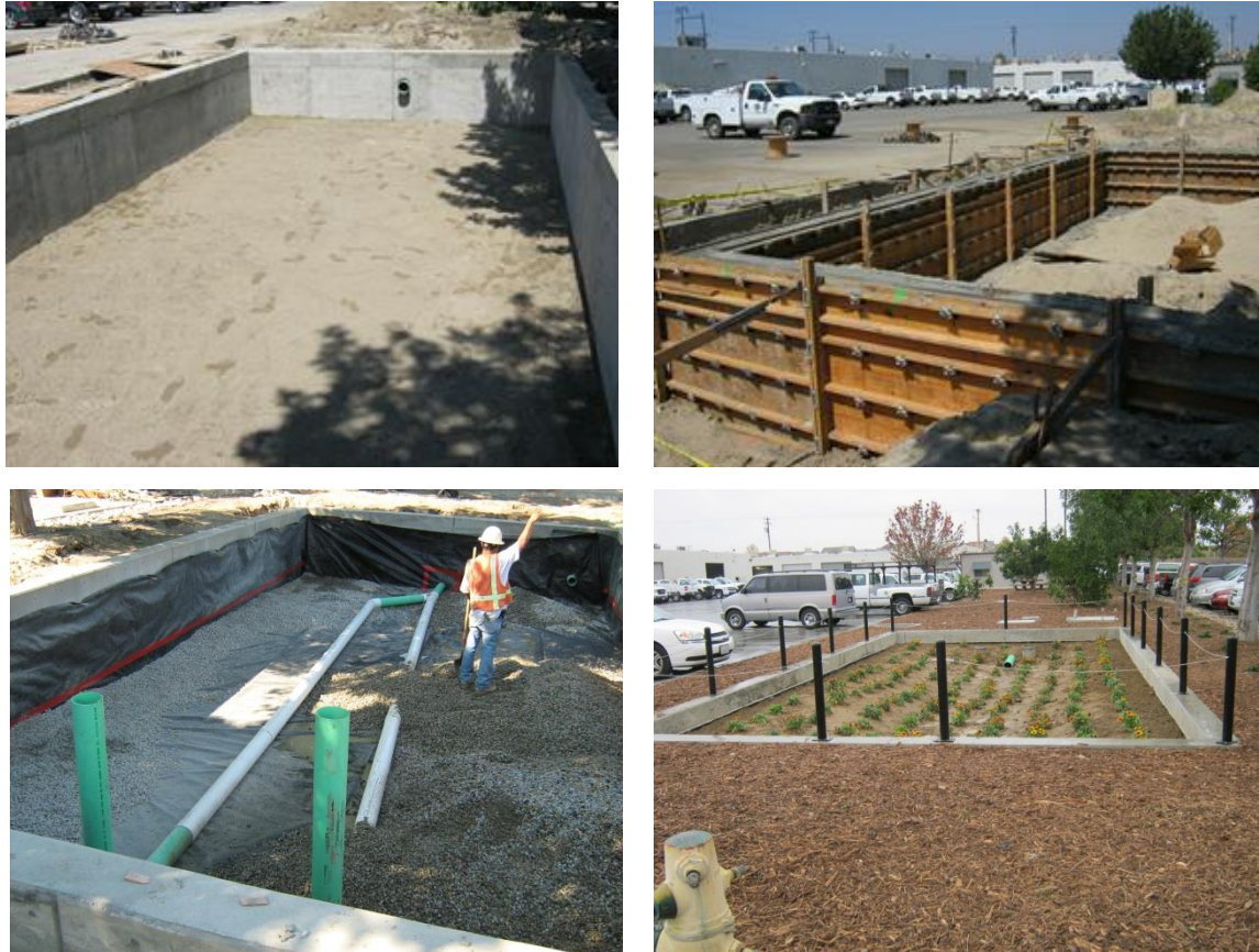
Figure 3-26. Photographs of Various Stages of Construction of a Bioretention Basin at LID BMP Monitoring Facility
